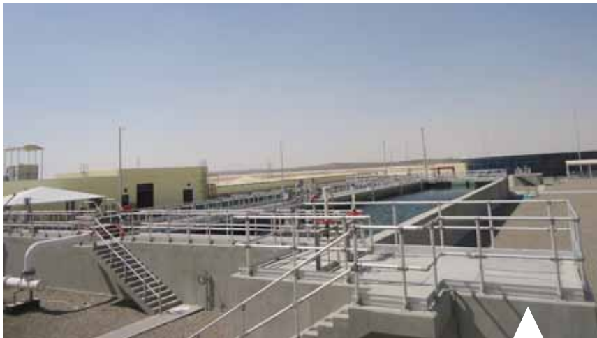
Waterzuiveringsstation, Razeen, Abu Dhabi, VAE
