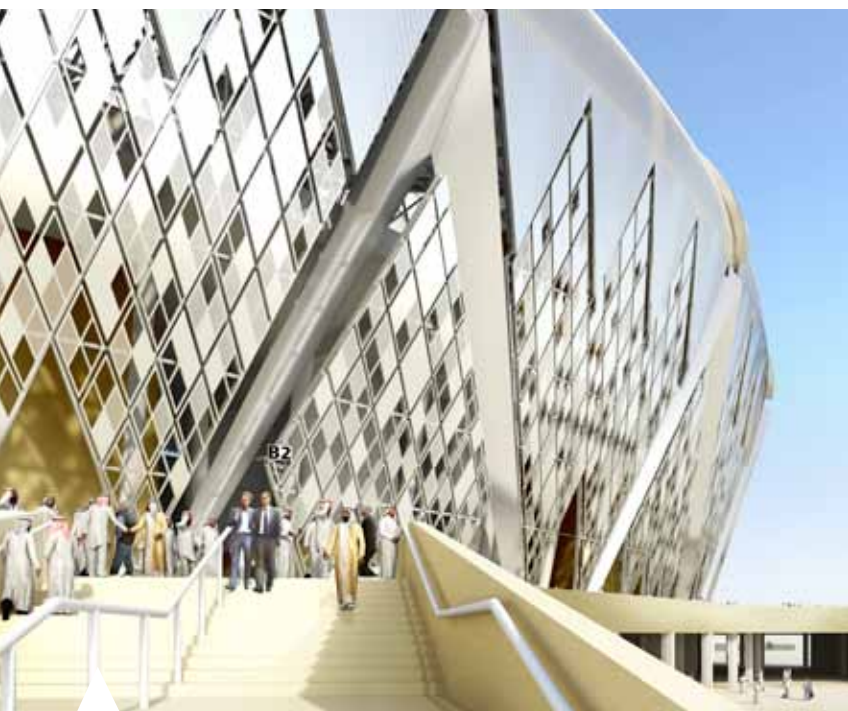
King Abdullah Sports City, Jeddah, Saoedi-Arabië Architect: Arup Associates
